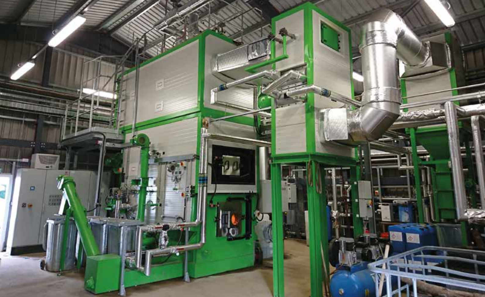
Biomass steam boiler at the Nc'nean distillery - Scotland's first net zero certified distillery utilising small roundwood from surrounding commercial plantations.
